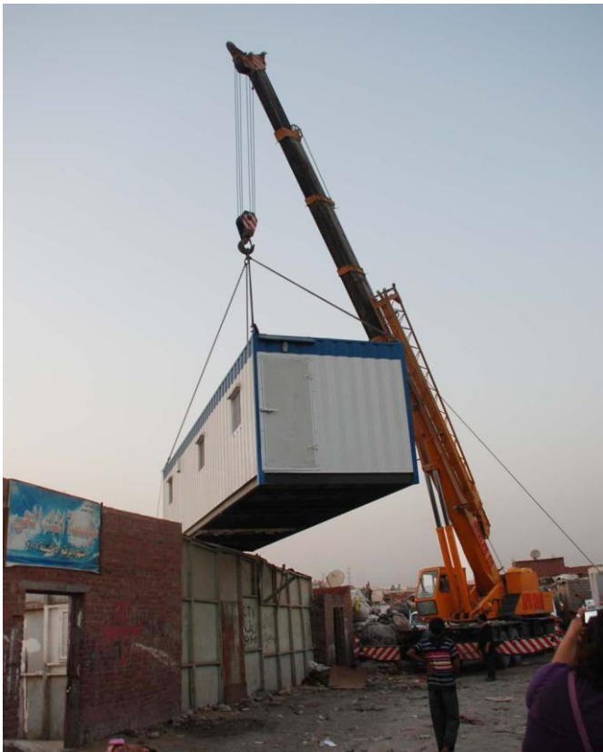
The crane brought the Container on its place in April 2013
